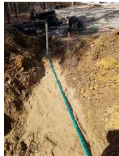
New Sewer service installed on Campo Lane
