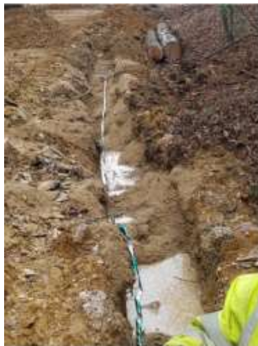
New Sewer service installed on Campo Lane
