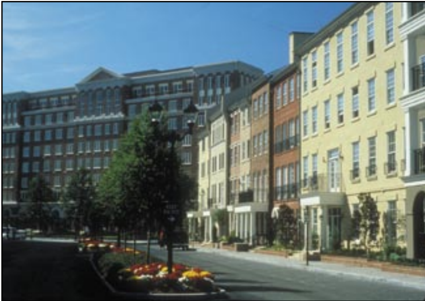
Riverside Village mixed-use project built for Post Properties in Atlanta. Office building, rear, is 226,000 sf. (Photo: Steve Hinds)
