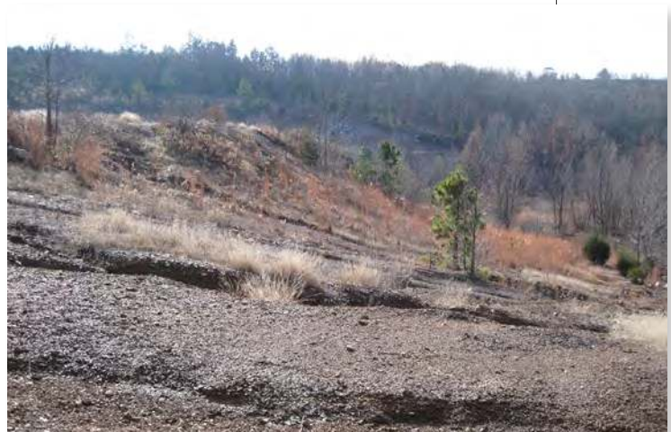
FIGURE 7.1. EROSION OF EMBANKMENT WITH POOR COVER
