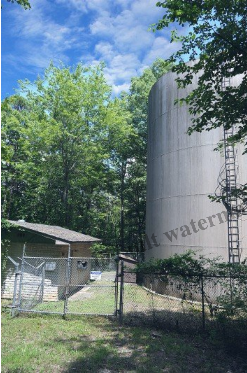
HSVPOA Water Tower Affected by Water Main Break
