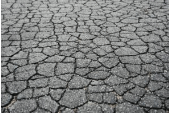
Example of alligator cracking (photo is NOT from HSV and is for illustrative purposes, only)
