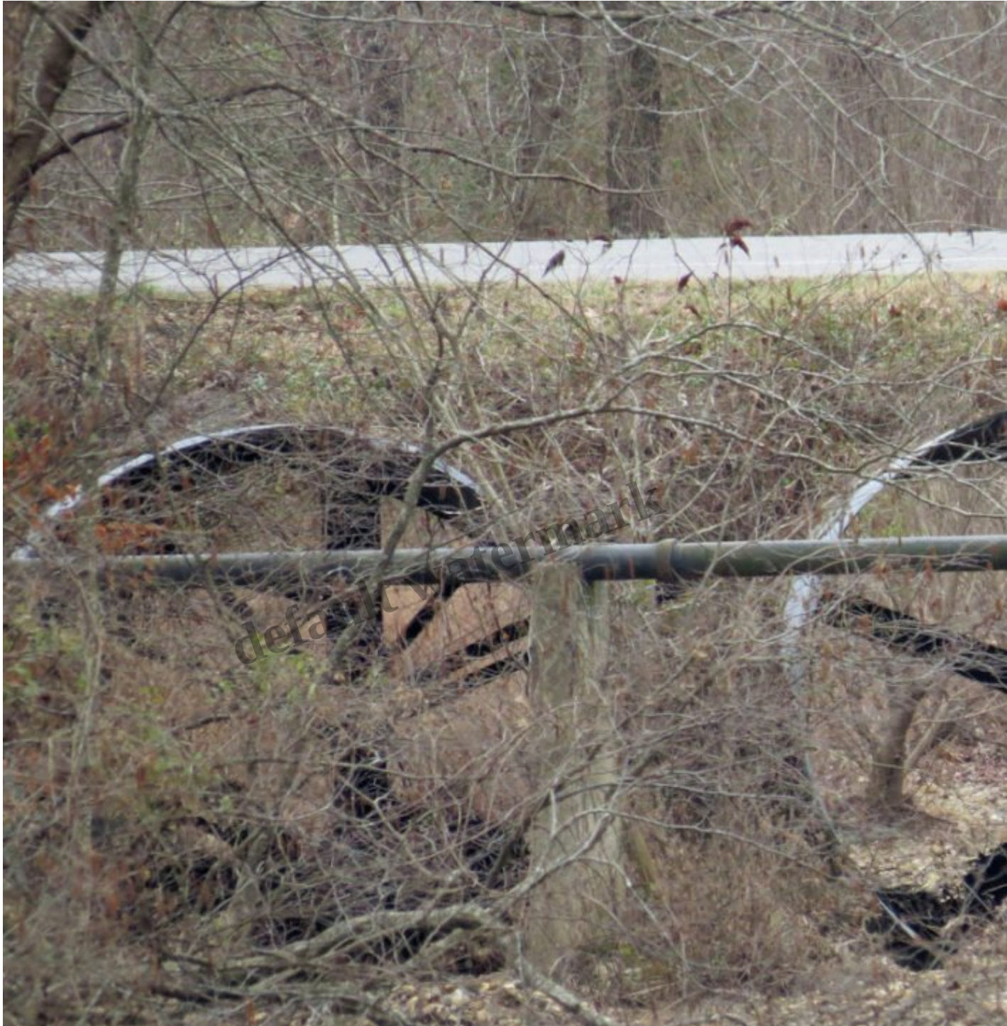
Hot Springs Village Culvert
