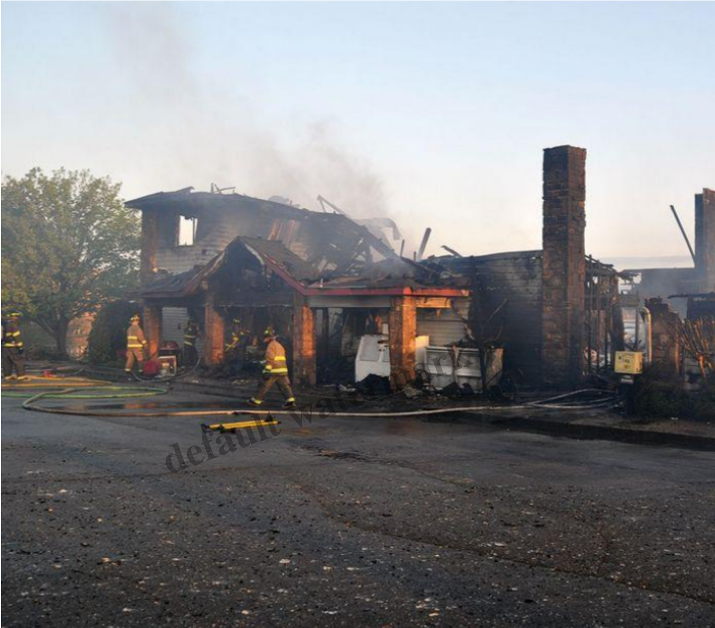
Balboa Marina Destroyed (photo courtesy of Hot Springs Village Voice Newspaper)
